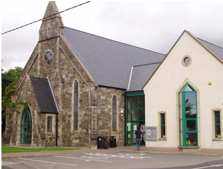
Figure 1. Former 19 th Century Presbyterian Church in Buncrana, Co. Donegal which has been refurbished and extended to accommodate the public library.
